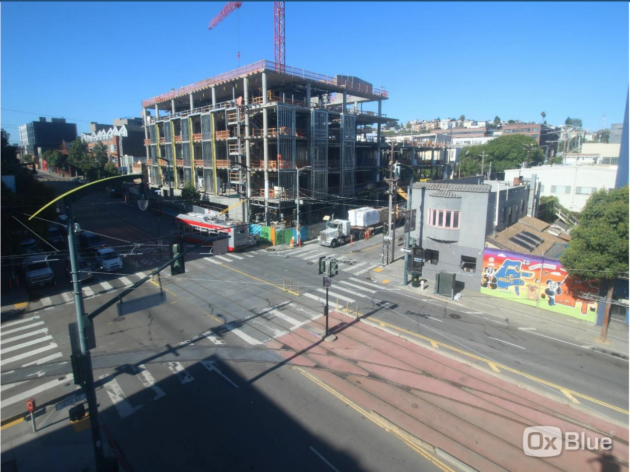
2130 Third Street – View from 3 rd & 18 th Street
