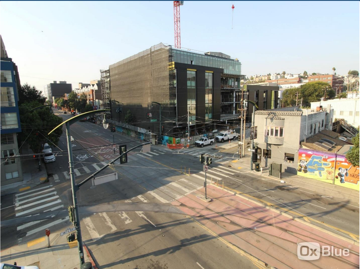
2130 Third Street – View from 3 rd & 18 th Street
